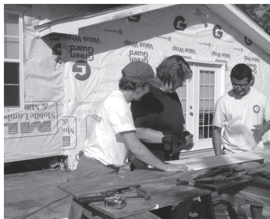
Parishioners help rebuild homes in Pass Christian, Mississippi.
